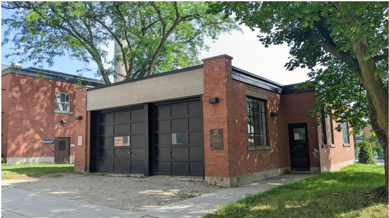
Blackwood and Old Firehall Studio Buildings
