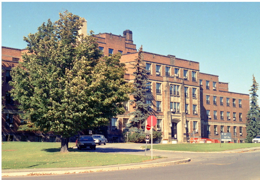
Figure 1. South entrance of K.W. Neatby Building, Ottawa. (Photo: J.E. O'Hara.)
